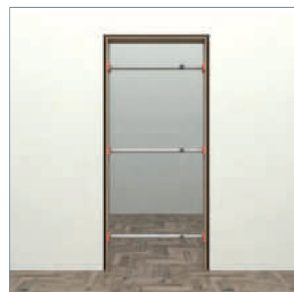
1. Set up the frame and brace it.
